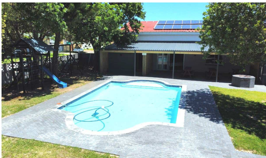
Carpark and Pool Area upgrades at the German Club.
